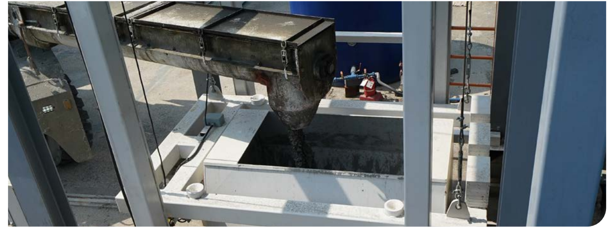
Step 5 Flying bucket concrete pouring
