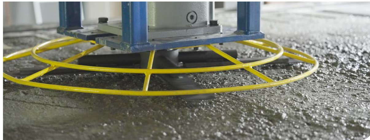
Step 9 Rotary surface finishing
