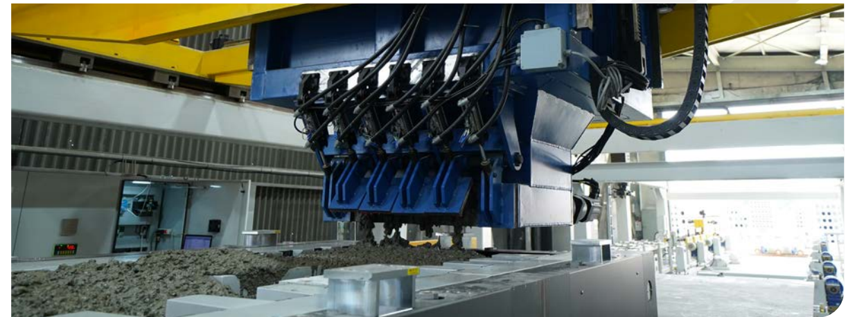
Step 6 Concrete distributor installation
