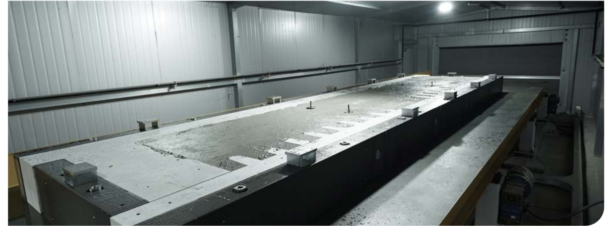
Step 11 Tunnel-type curing chamber operation
