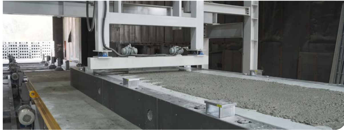
Step 8 Screed surface finishing
