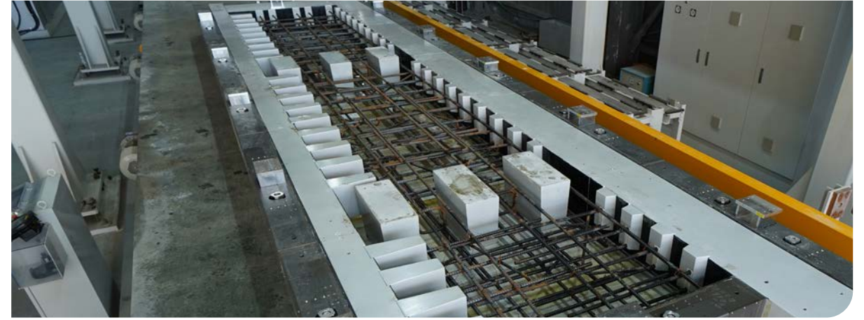
Step 4 Mold positioning and setting
